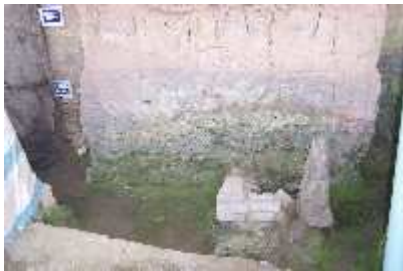
Pavilion pillar base of compacted gravel
